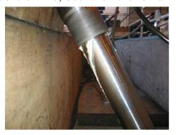
pumped through we got a pressure increase an the valve opened. Some more *Enviroseal* was pumped and we registered 400 bat at the control line. We keep the pressure on for 20 minutes, an bled it off very carefully and the valve closed. We opened and closed the valve 6 times. Everything looked very fine.
